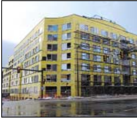
Manchester Place under construction
