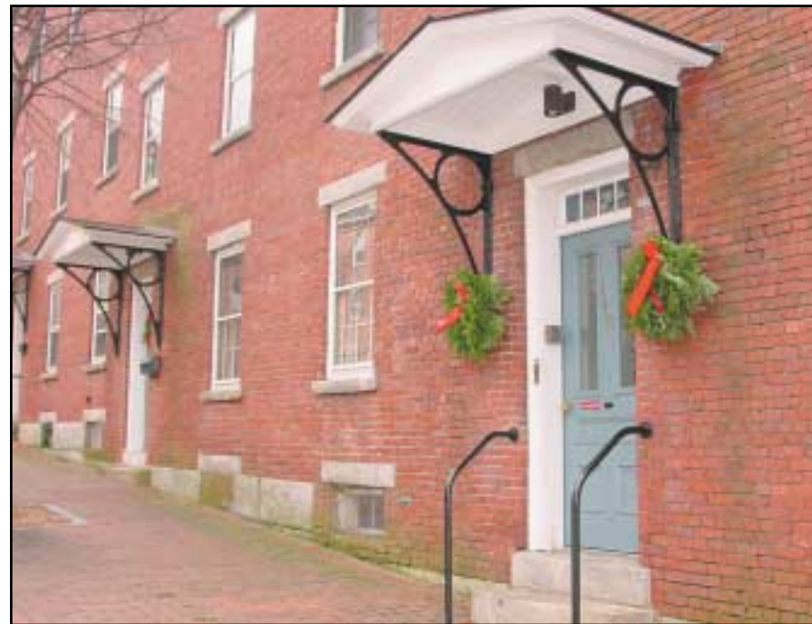
Residential units built in the 19th century for mill workers are desirable housing for 21st century urbanites
