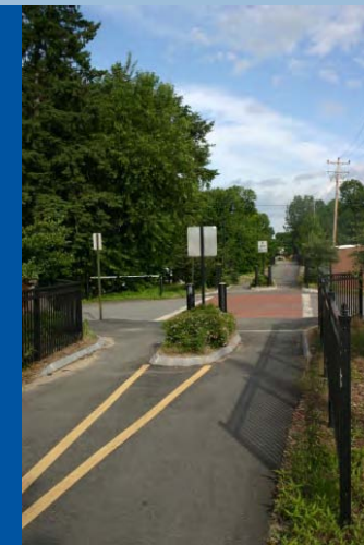
Section of the Piscataquog Trail crossing Third Street
