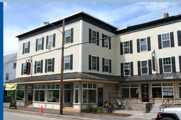
A redeveloped mixed use building in a mixed use neighborhood (Rimmon Heights)
