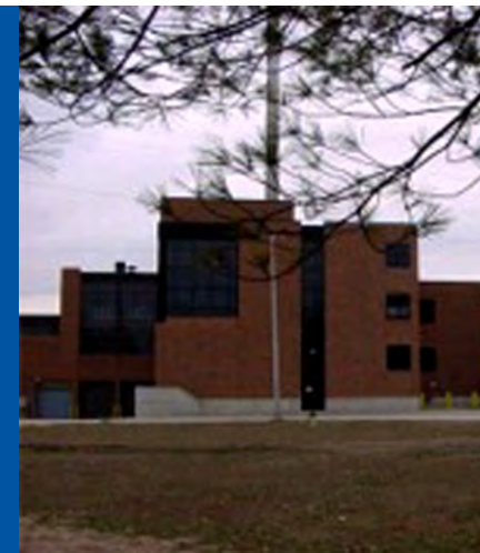
The Wastewater Treatment Facility on Gay Street
