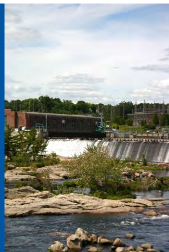
Amoskeag Hydro station, one of two hydro facilities in the City providing clean alternative energy
