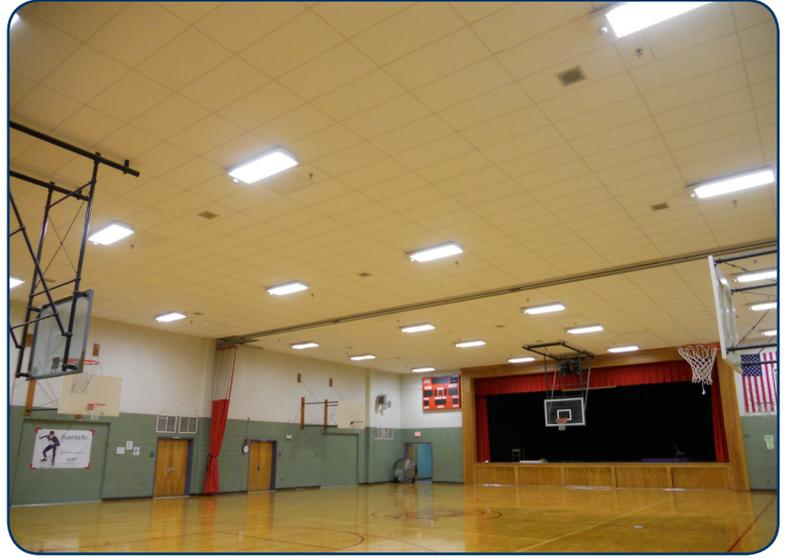
Each light fixture has a motion sensor, when the gym is unoccupied, the light will automatically turn “off” after an adjustable time delay.
